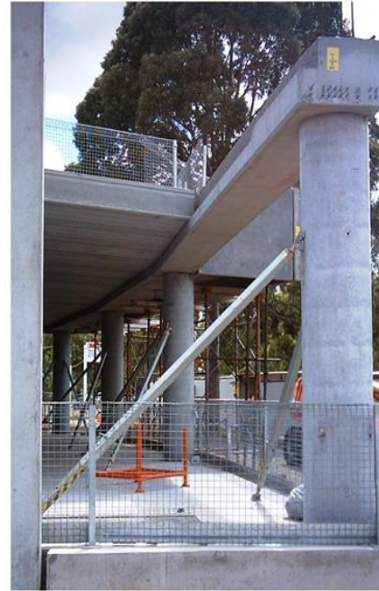
Description: Precast reinforced concrete columns, beams and slab panels.
