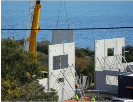
Description: Precast concrete panel system for housing Source: By courtesy of Mark Vines of RMIT University
